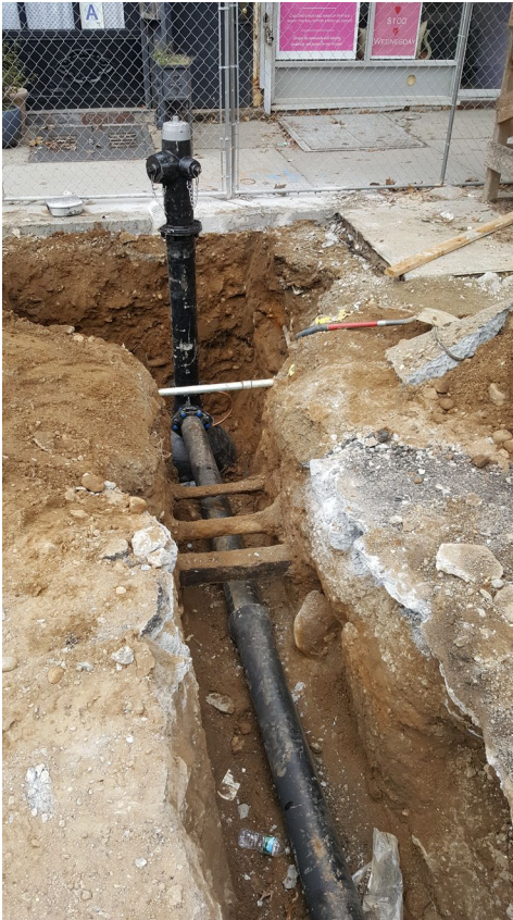
New hydrant installed on Putnam Avenue
